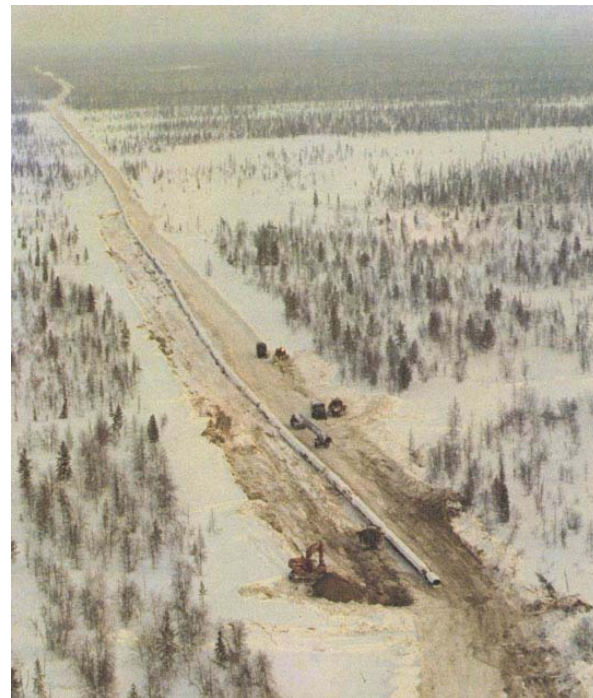
Construction of a gas pipeline, Siberia.
